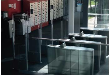
In addition to the kiosks, one book sorter was installed at each of the main libraries. The sorters are specially designed to be both quiet and extremely economical while still allowing for fast and accurate sorting of library materials with very little need for staff intervention. The modular design of the sorters makes them an extremely flexible solution and means it is possible to build a system to fit the space available.
